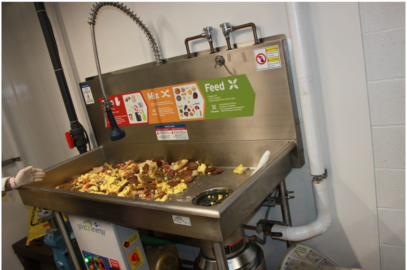
The system's grinder is designed to process most food waste, including meat, bones, and oils, and accepts both pre-consumer (kitchen scraps) and postconsumer (food waste returned on plates) food waste. Photo by Leah Graham.
