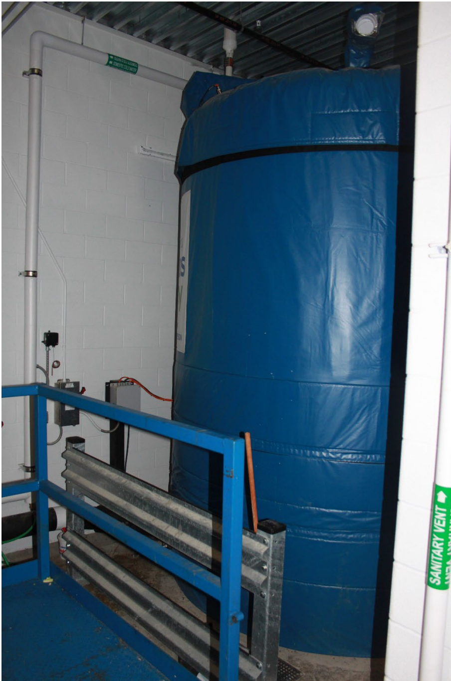
DI Hub's storage tank. The ground food is combined with water to make a slurry, which is pumped into the tank where it is stored without odors that could attract rodents and pests. When the tank is full, a third-party contractor pumps out the tank and transports the slurry to an off-site location for anaerobic digestion. Photo by Leah Graham.
