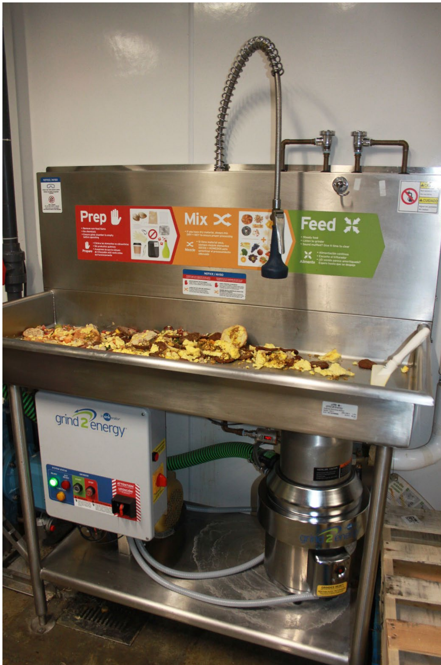
The system's grinder is designed to process most food waste, including meat, bones, and oils, and accepts both pre-consumer (kitchen scraps) and postconsumer (food waste returned on plates) food waste. Photo by Leah Graham.
