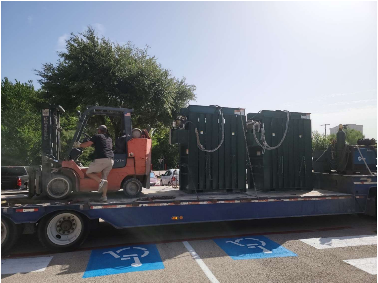
Picture 5. Day of baler installation on flatbed truck with forklift at Brookhaven Campus and North Lake Campus.
