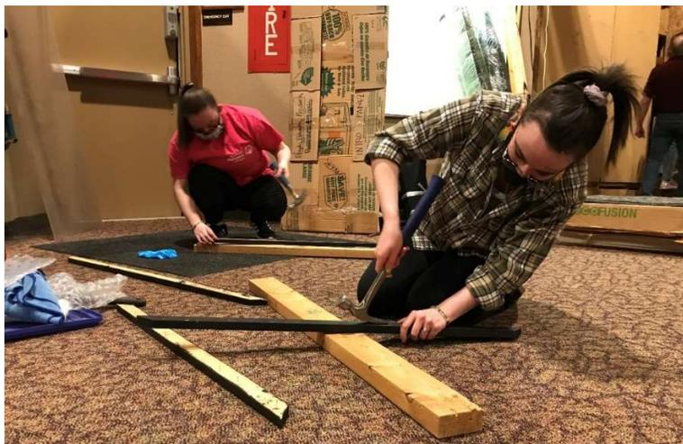
Extracting nails and screws so that both the wood and the fasteners could be reused was very laborious for Museum Studies students, but it made the success of the adaptive reuse possible.
