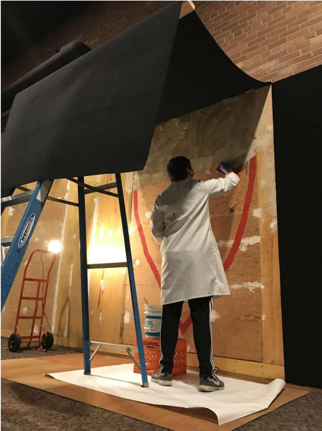
Salvaged 2x4s and plywood panels were used to clad the existing brick wall in the installation area and support the use of new inexpensive carpet to create a neutral exhibit backdrop. Those recycled materials are clearly visible beneath the carpet being installed by students. The autographed “heart” placed in the exhibit was intended to encourage future students to recycle the same material. Hopefully this will create a tradition among CMU Museum Studies students.
